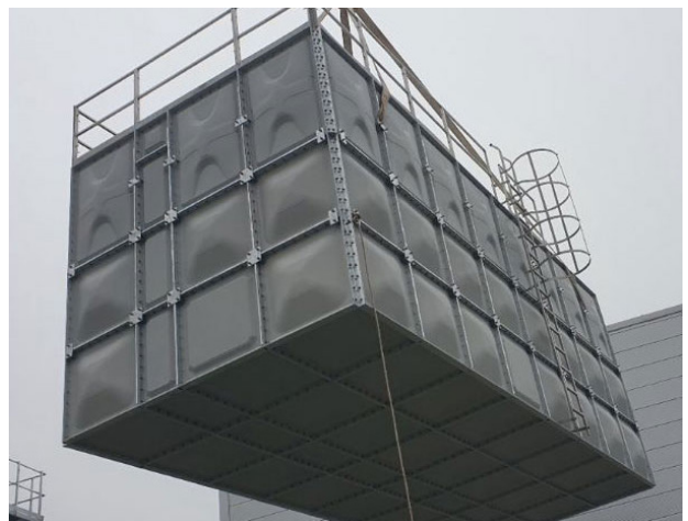
Final GRP Tank placement
