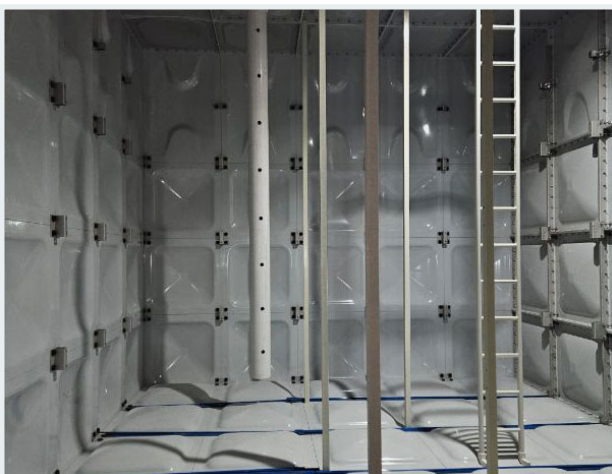
Roof & support assembly
